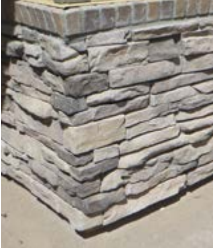
Veneer close to slab as possible example
