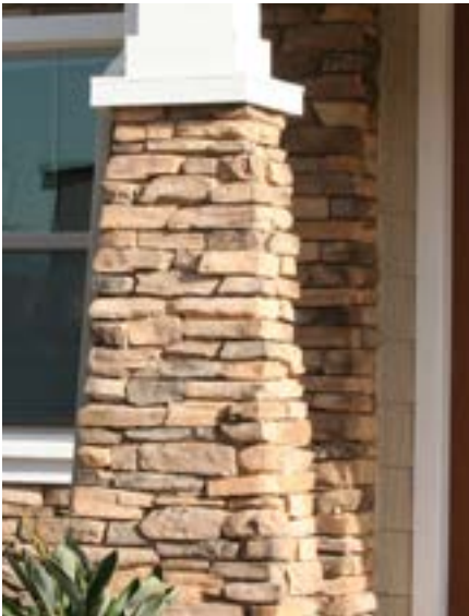
Examples of veneers wrapping columns entirely
