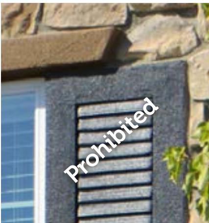
Example of prohibited embedded shutter
