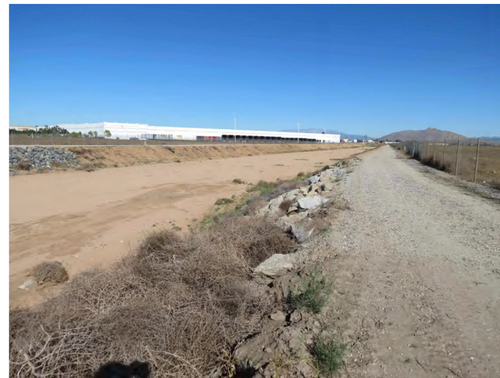
Photograph 8: View looking within the Perris Valley Storm Drain. Photo taken March 26, 2015.
