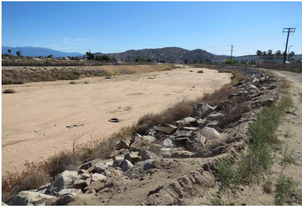
Photograph 1: Photograph depicting the Perris Valley Storm Drain.
