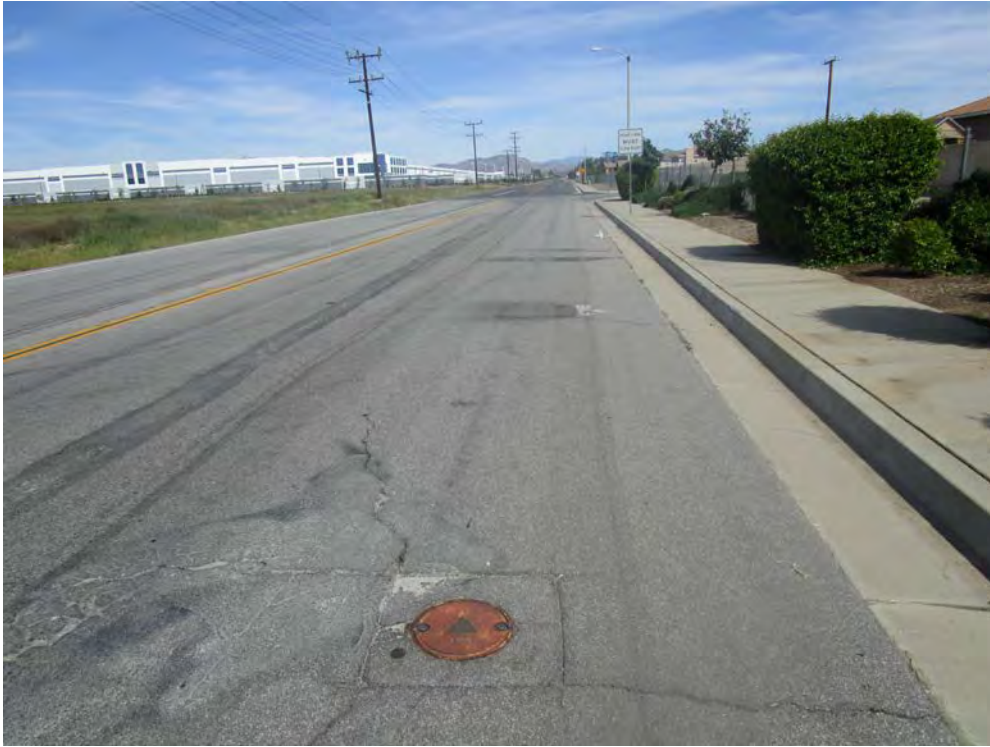
Photograph 11: Both monitoring wells on Indian Street.
