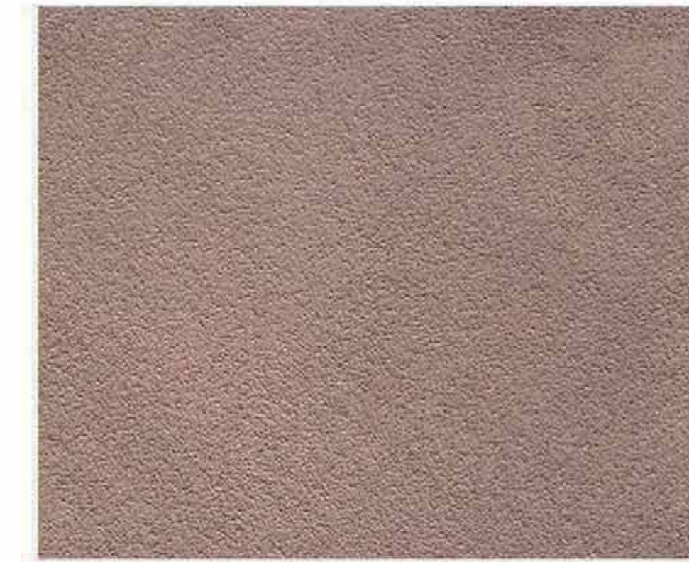
Trash Enclosure Wall Stucco Finish Spanish Texture
