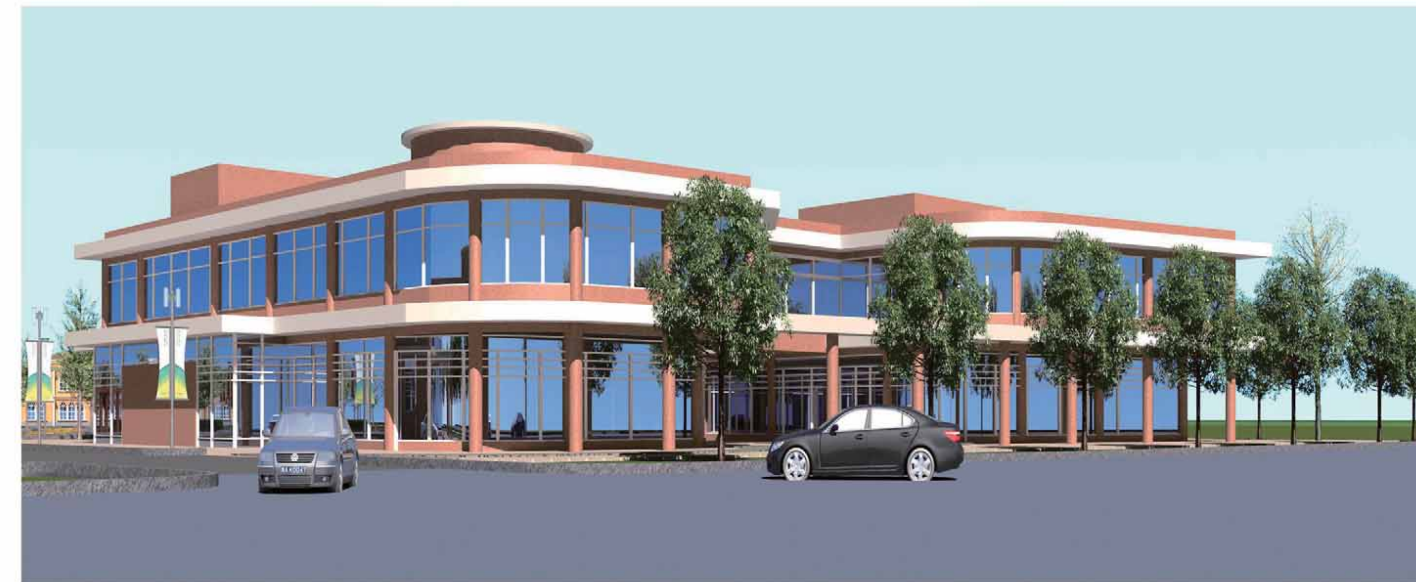
Nason Street Southwest and Northwest Corners
