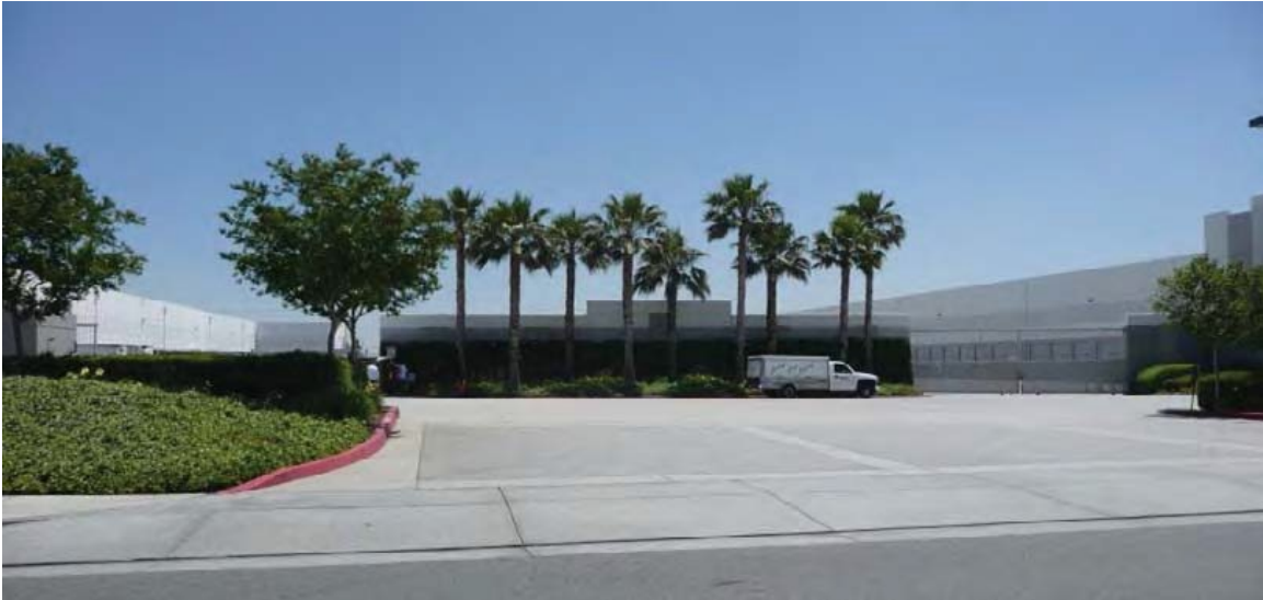
Figure 5-25 Example of Appropriate Ground Mounted Equipment Screening
