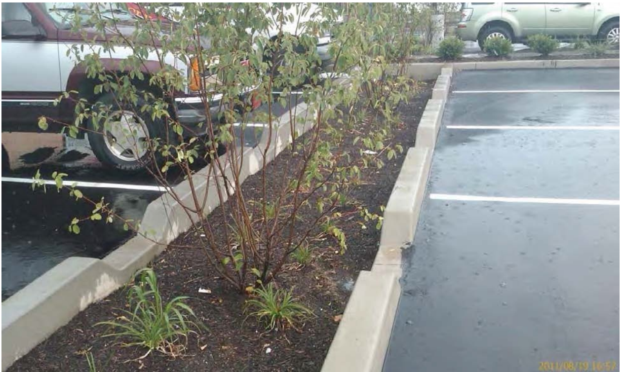
Figure 5-35 Example of Bio-swale
