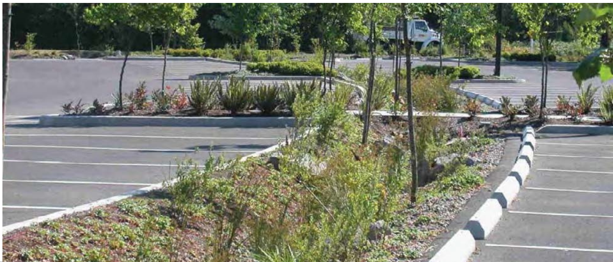
Figure 5-7 Example of Biodetention Facility
