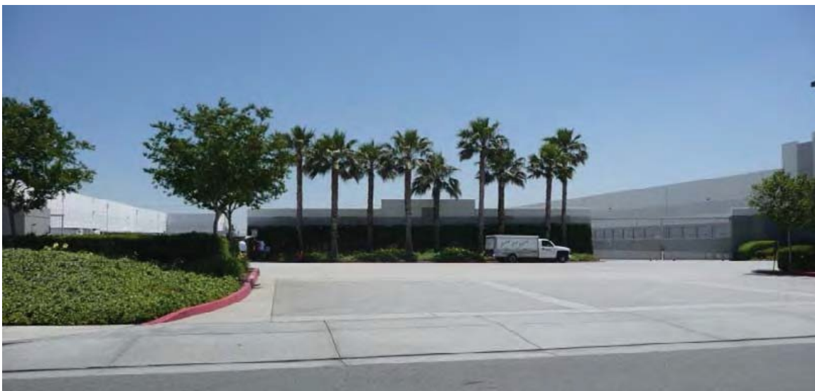
Figure 5-25 Example of Appropriate Ground Mounted Equipment Screening
