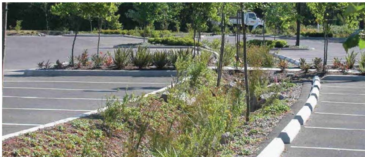
Figure 5-7 Example of Biodetention Facility
