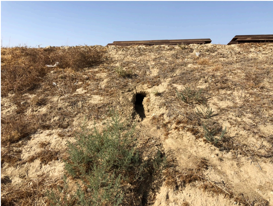
Photo 2 – 2 nd of 2 burrows observed, looking north from bottom of storm water catch basin.
