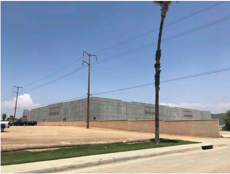
View of Adjacent Bldg Under Construction
