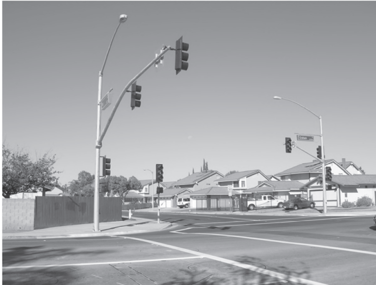
Traffic Signal and Street Improvements at Graham St and Bay Ave
