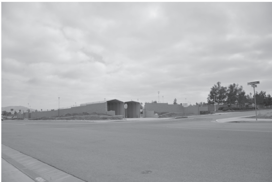
Public Safety Building Parking Lot Expansion
