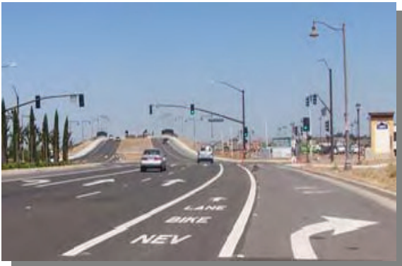
NEV/Bike Lane Pavement Marking and Striping in Lincoln, CA
