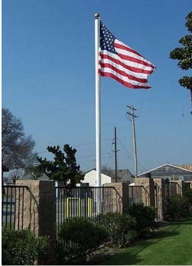
Example of Telecommunication Tower in Flag Pole
