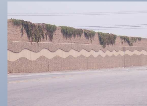
Local Street side
