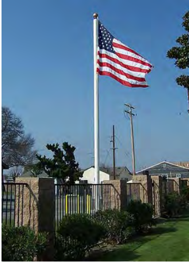
Example of Telecommunication Tower in Flag Pole
