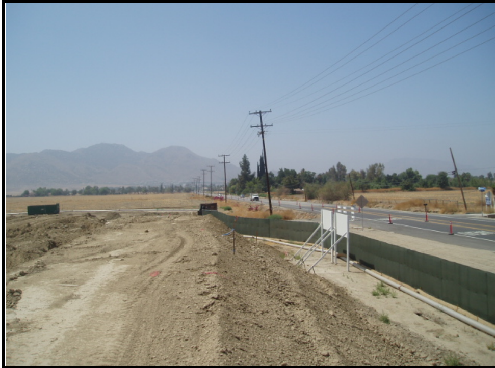
LOOKING SOUTH ALONG REDLANDS BOULEVARD
