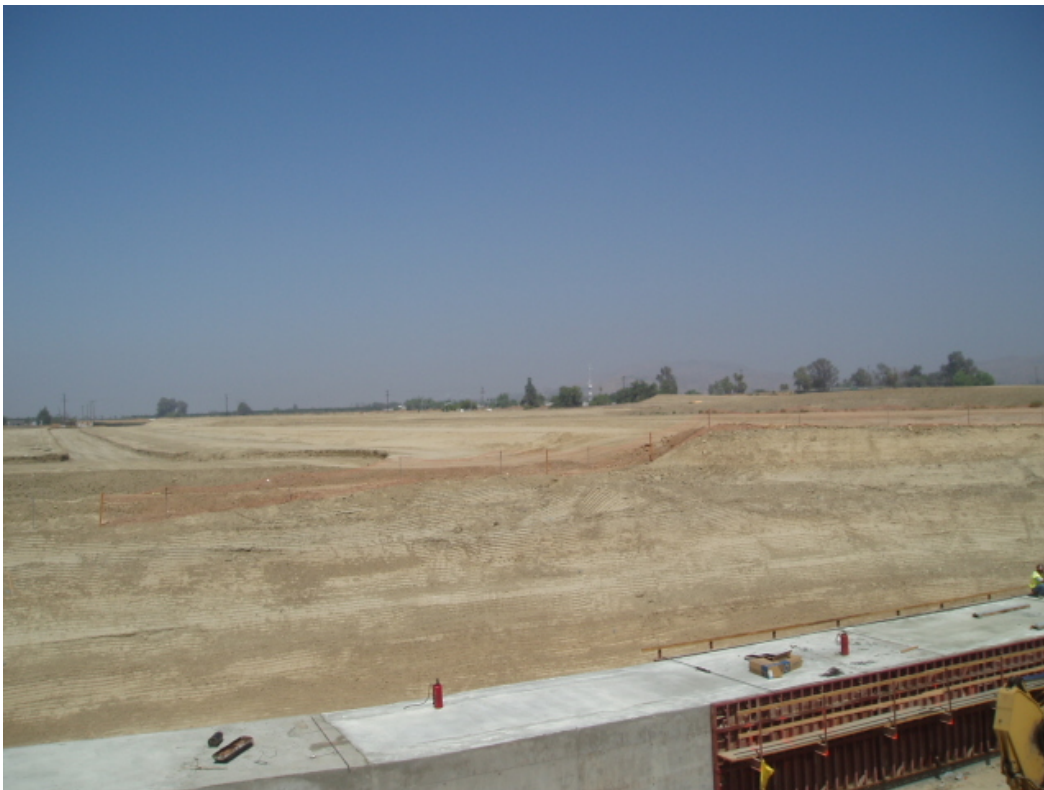
VIEW OF PARCELS 2 & 3 FROM SOUTHEAST
