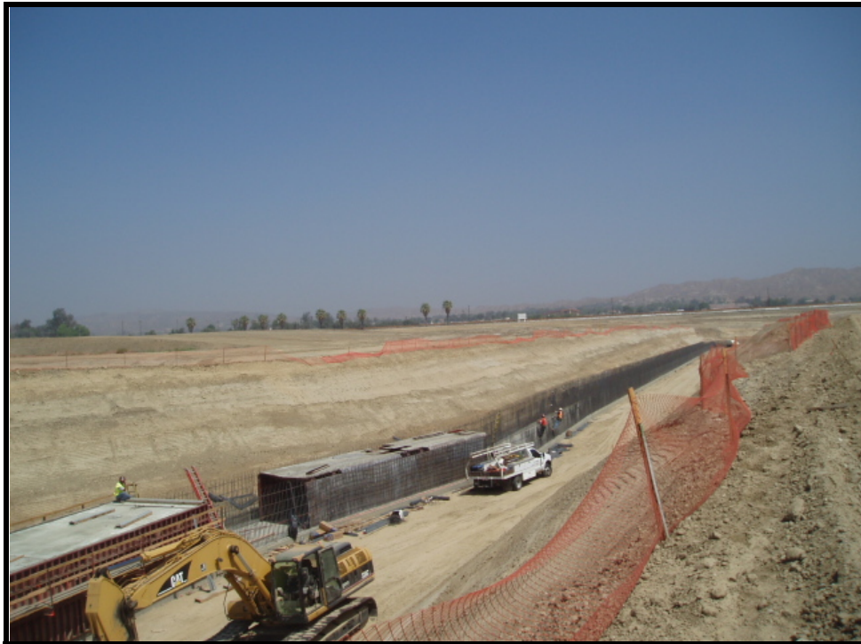
STORM DRAIN UNDER CONSTRUCTION
