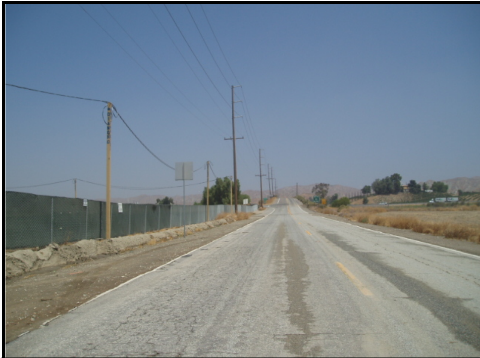
LOOKING NORTH ALONG THEODORE AVENUE
