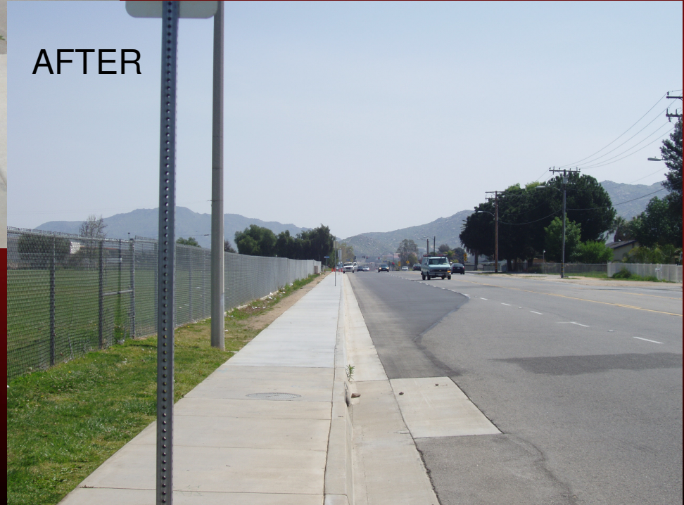
Iris Avenue from Indian Street to Perris Boulevard
