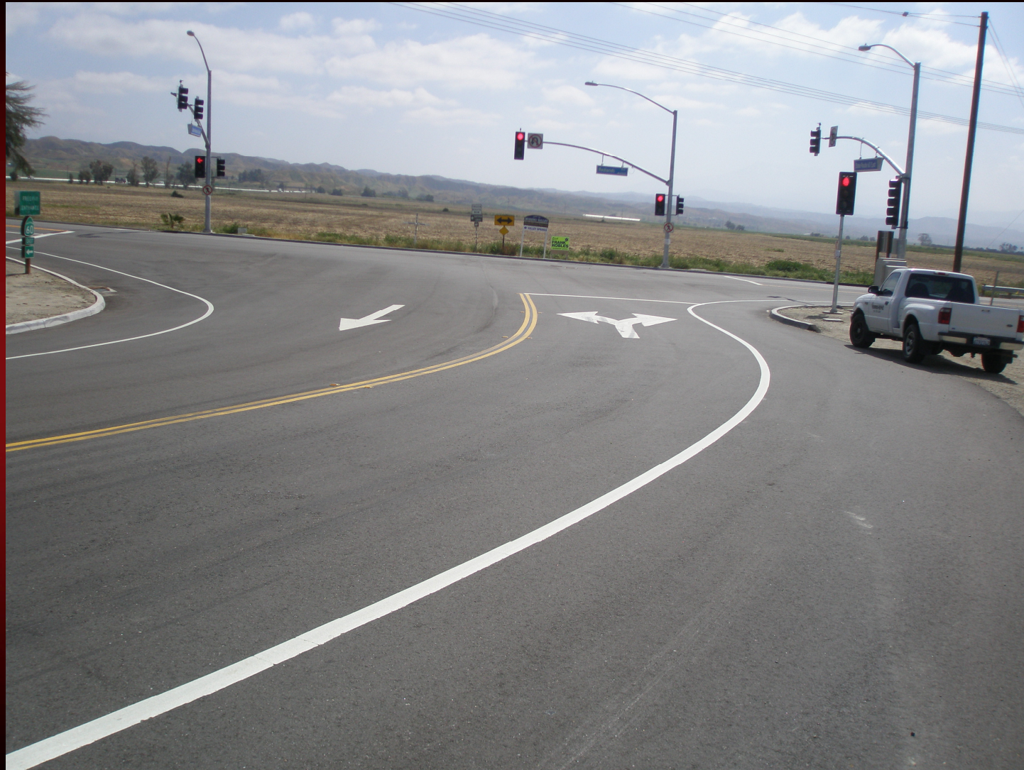
SR-60 Eastbound Ramps / Redlands Boulevard Traffic Signal
