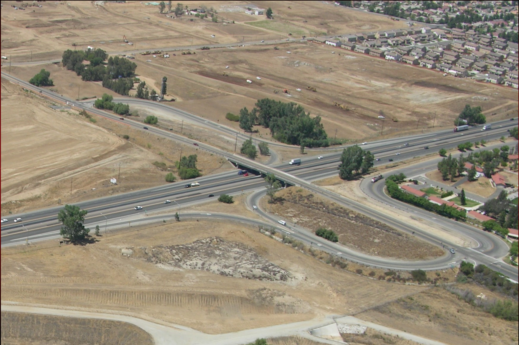
SR-60 / Nason Street Interchange
