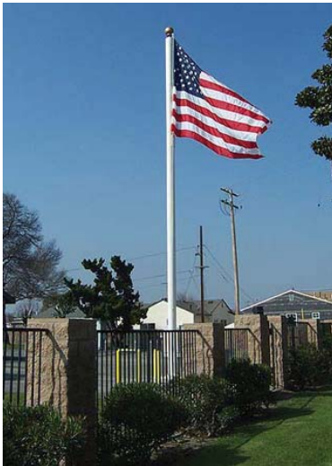
Example of Telecommunication Tower in Flag Pole
