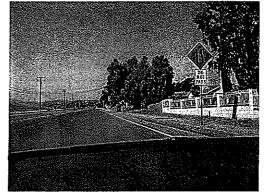
• Curb returns at the Alessandro intersection do not appear to come close to accommodating ultimate design (subject to additional traffic analysis). Actual returns would need to be constructed and signal would need to be analyzed to see if it needs to be relocated.
