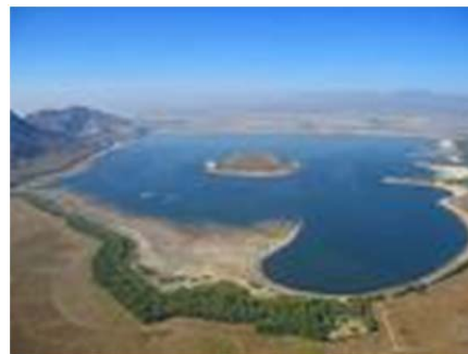
Figure 12-1: Perris Dam Construction Project 39
