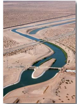
Water conserved by the All-American Canal Lining Project is an important part of the Water Authority's Colorado River water transfer supplies.
