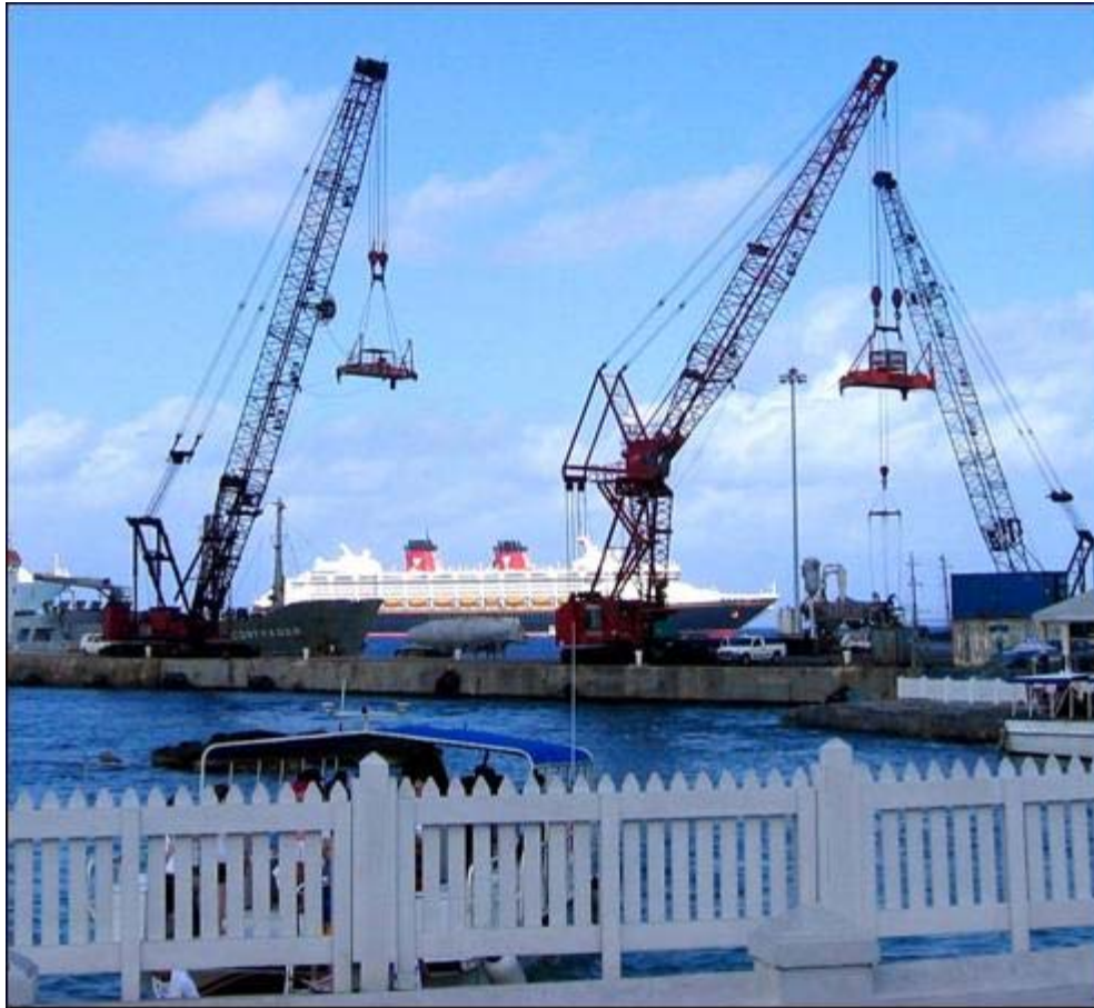
Figure 3.4 Construction in paradise (Photo #1033)
