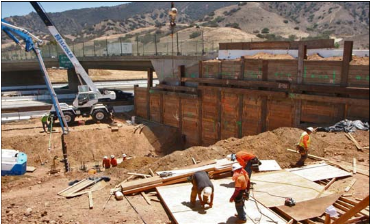
Green River Road / SR-91 Interchange construction (Photo courtesy of RCTC)
