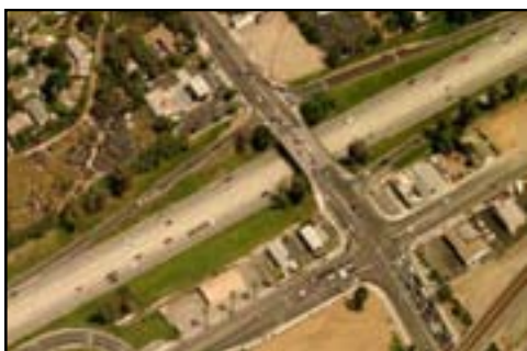
Van Buren / SR-91 Interchange Project, City of Riverside (Photo courtesy of City of Riverside)
