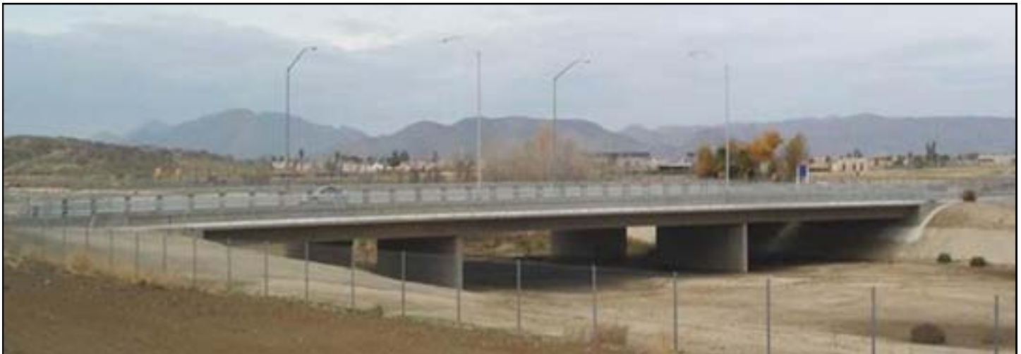
Sanderson Avenue Bridge Project over Salt Creek, City of Hemet (Photo courtesy of City of Hemet)
