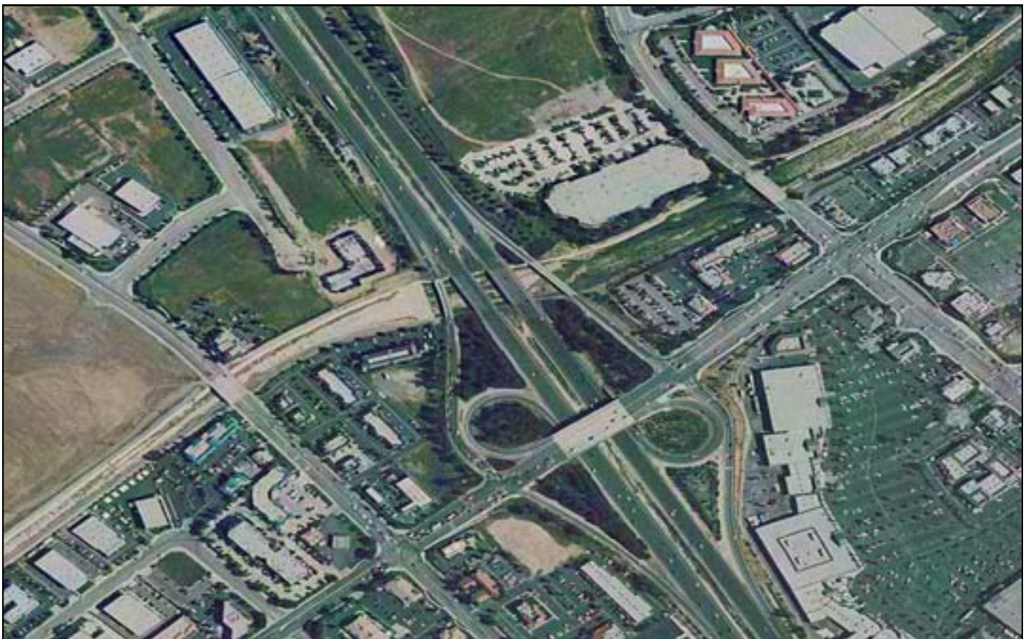
SR-79 Winchester Road / I-15 Interchange Project, City of Temecula (Photo courtesy of City of Temecula)
