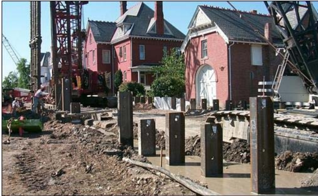
Figure 3.1 Construction in residential area (Photo #924)
