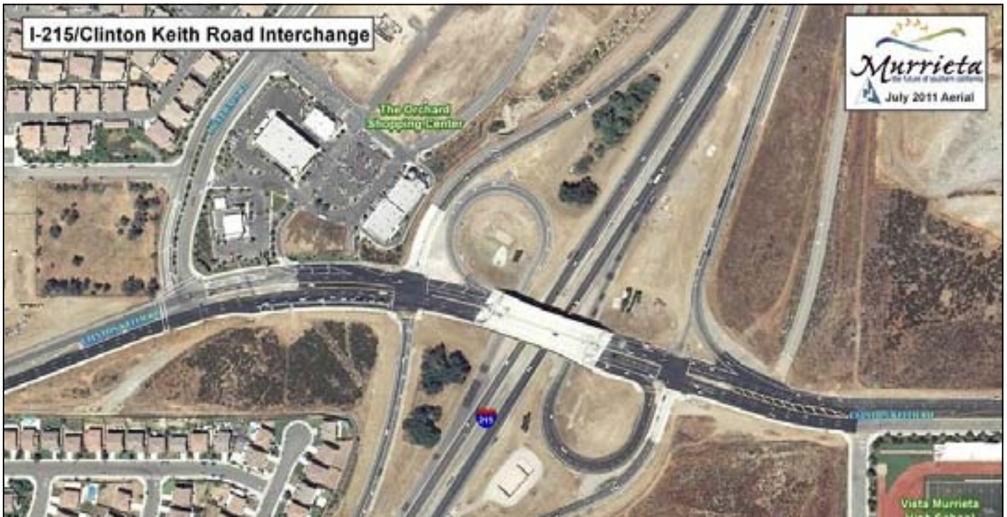
I-215 / Clinton Keith Road Interchange Project, City of Murrieta (After improvements) (Photo courtesy City of Murrieta)
