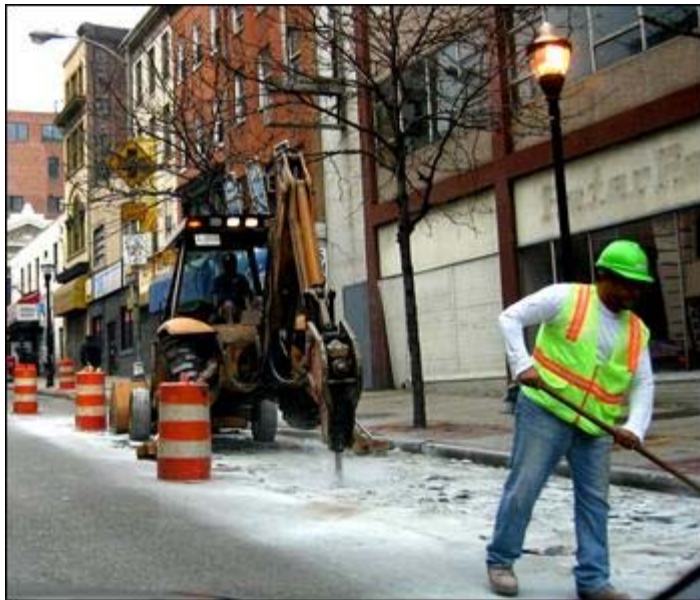
Figure 3.2 Construction in business district (Photo #714)
