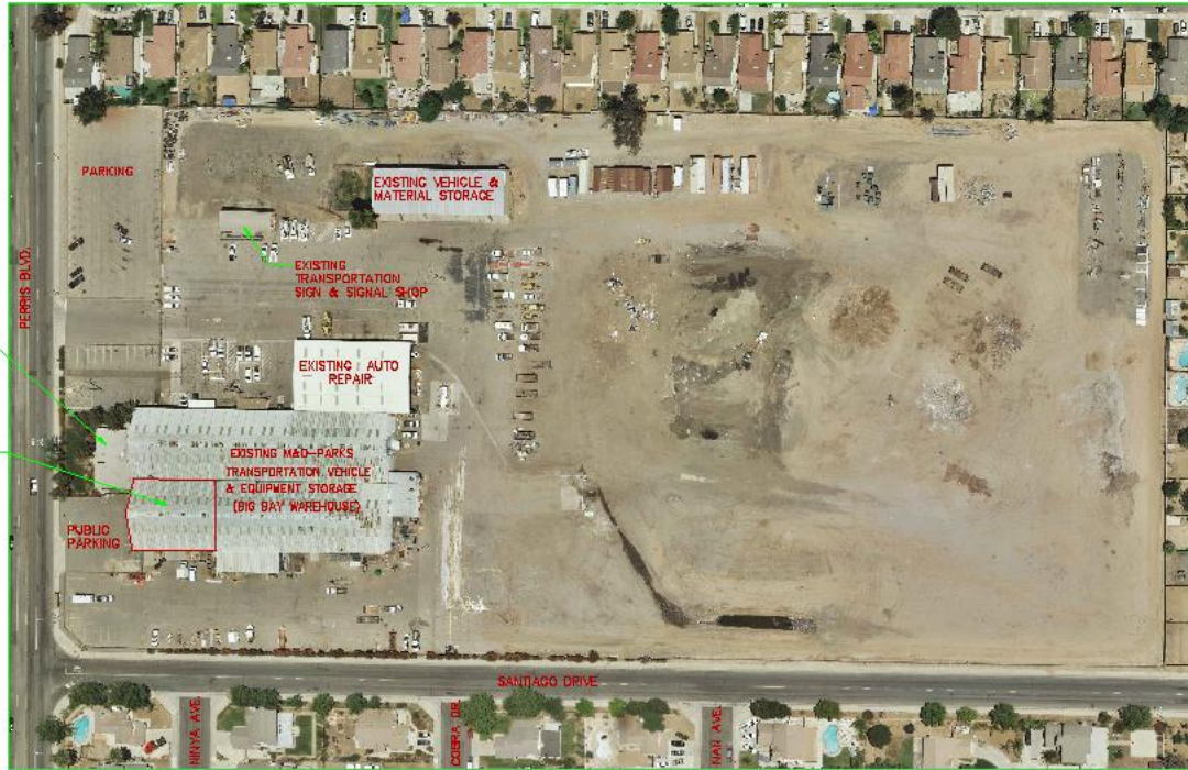
EXISTING SITE CONDITION
