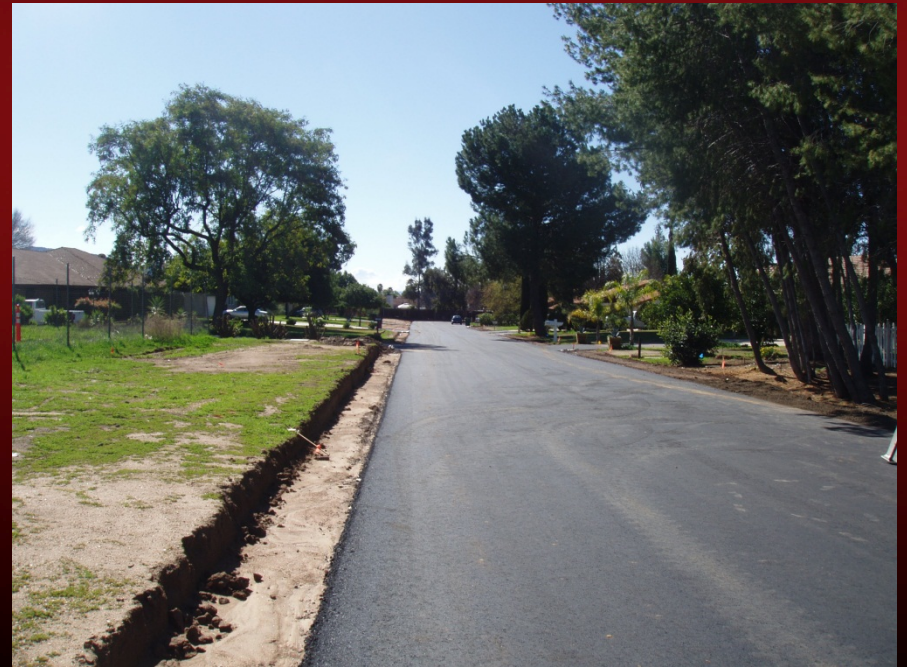
Kentland Lane AFTER
