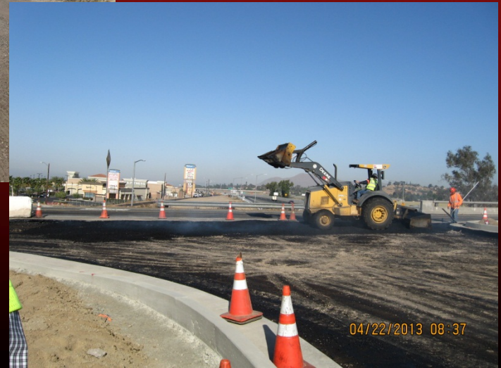
SR-60 / Moreno Beach Drive South Side of Interchange (Phase 1)
