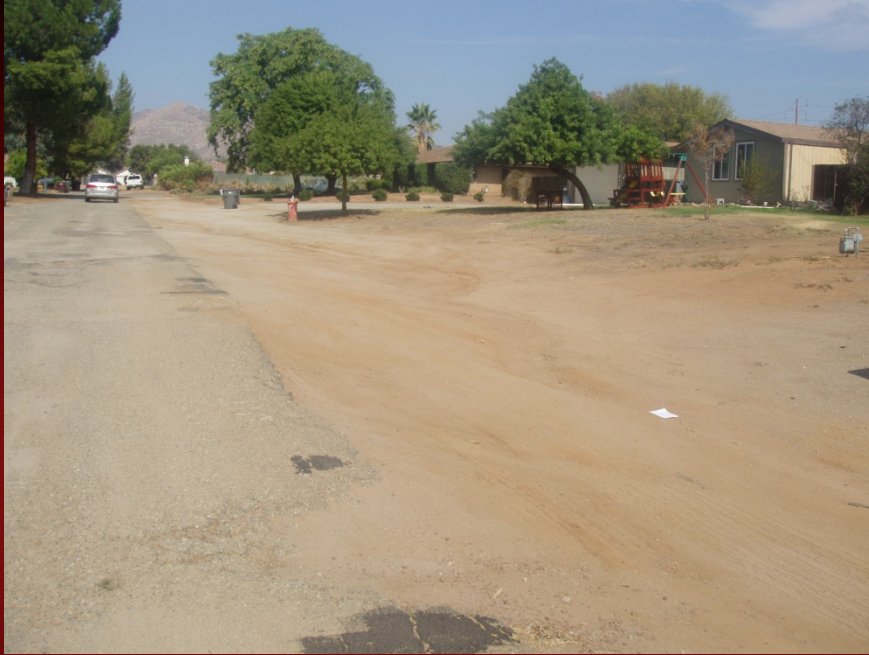
Kentland Lane BEFORE
