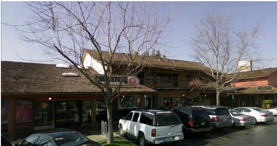
Fig Gardens: Walkable commercial community center.
