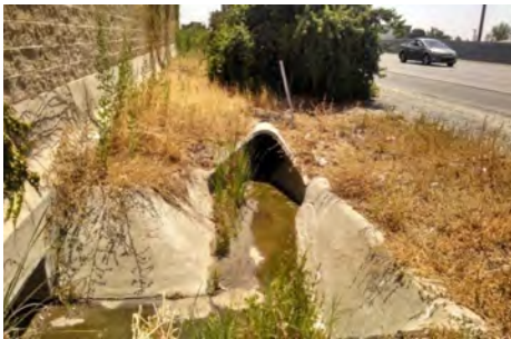
Figure 3. Existing pipe inlet
