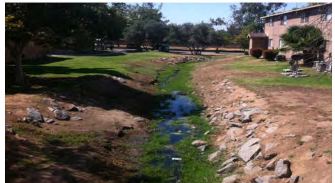
Line F open channel through Towngate Racquet Club Apartments
