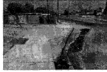
PONDING ISSUE SIDEWALK / CURB TRANSITION
