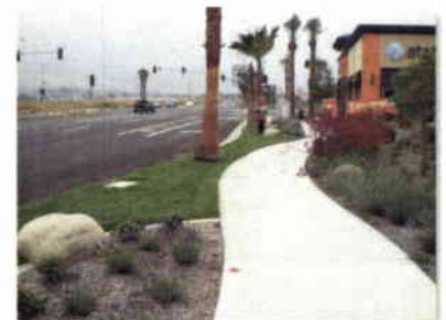
Parsons Brinckerhoff provided engineering design for new paving and lighting along Greenspot Road.
