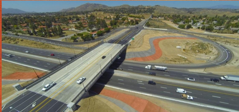
SR-60 / Nason Street Overcrossing Bridge
