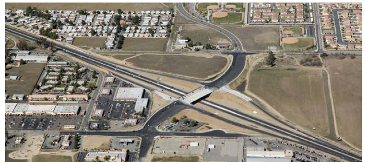
SR-74 / 4th Street / I-215 Interchange, City of Perris and RCTC. (Photo courtesy Skyview Imaging)
