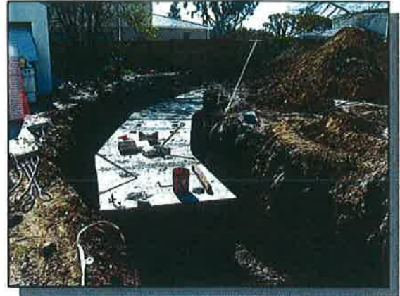
Downstream portion of 6.0'Wx3.5'H Reinforced Concrete Box
