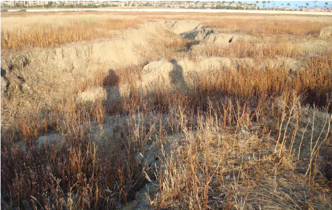
Eroded channel on the western portion of the project site.
