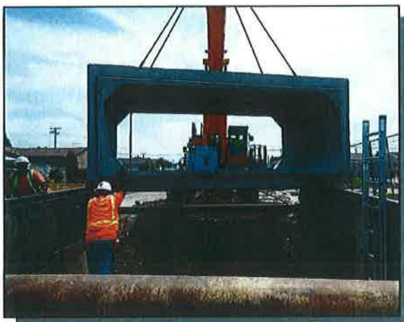
Reinforced Concrete Box
