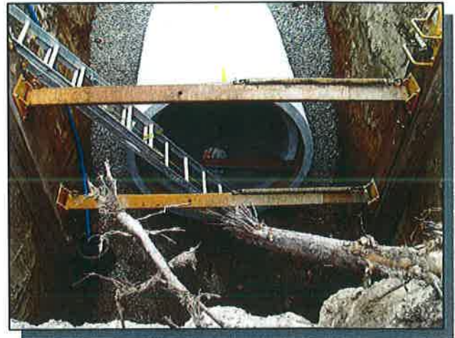
Electric Avenue Storm Drain
