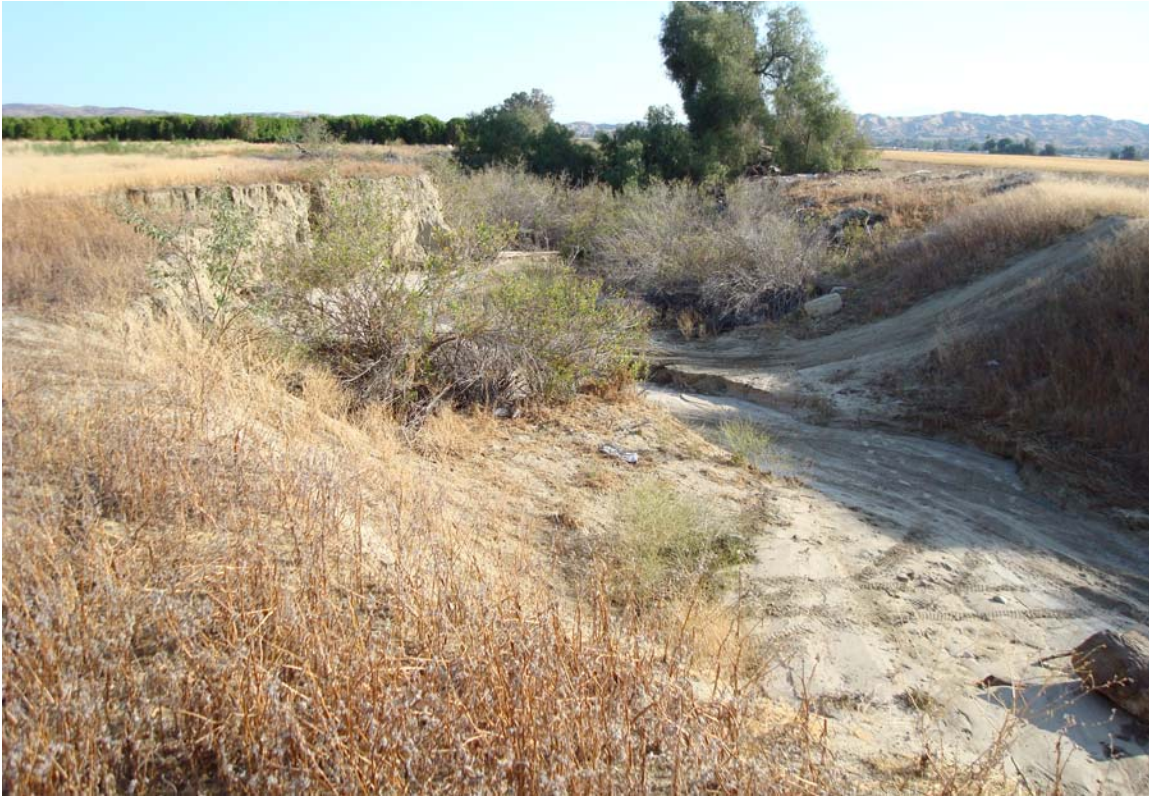
Southern portion of the eastern drainage channel.
