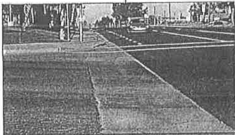
PHOTO 3 | Intersection reprofiling will require removal of existing cross-gutters
