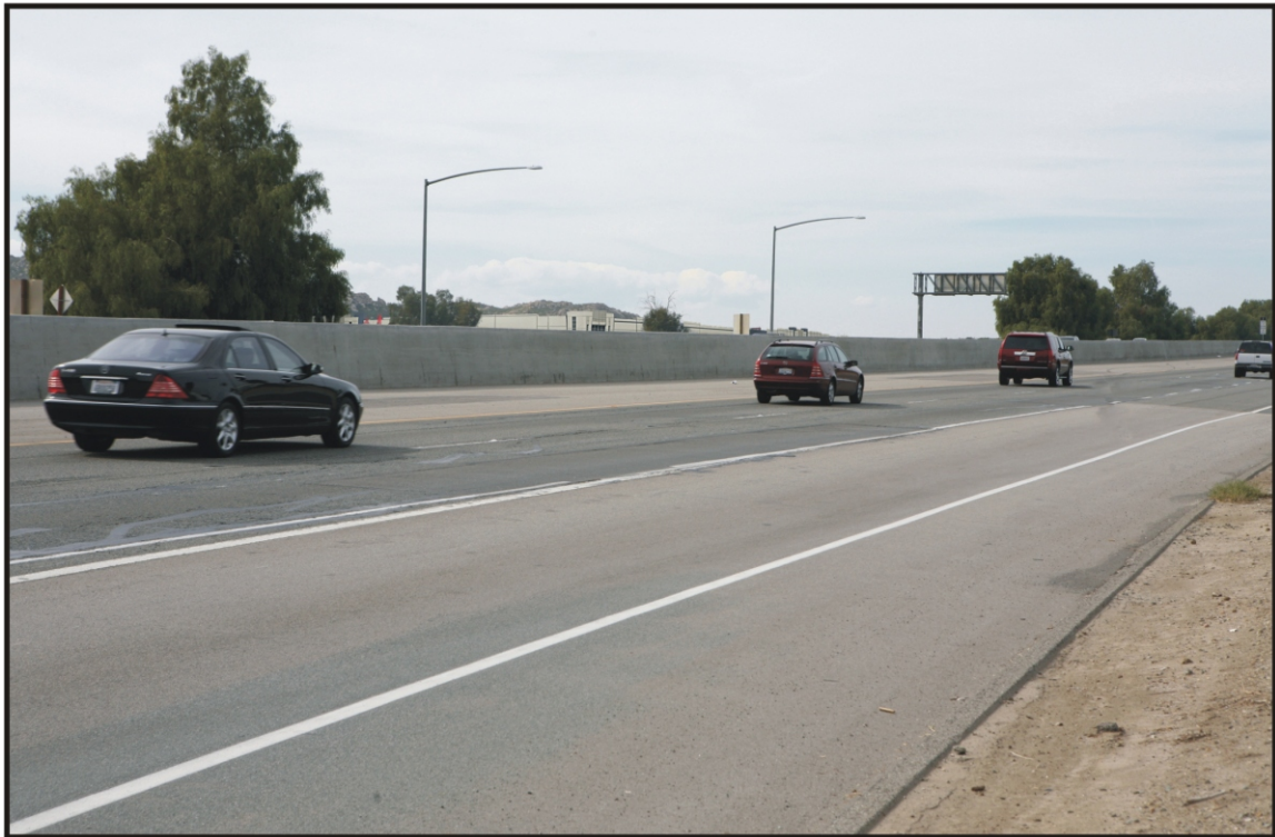
Project Buildout Condition
