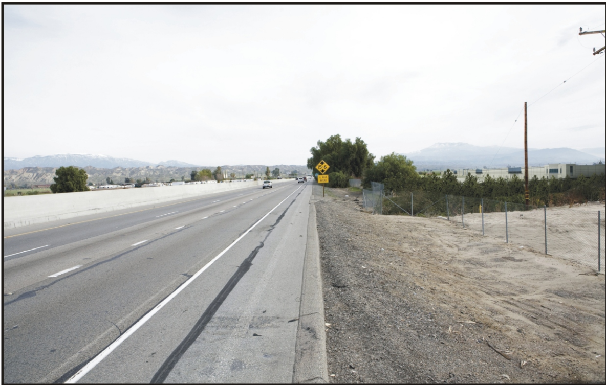
Project Buildout Condition
