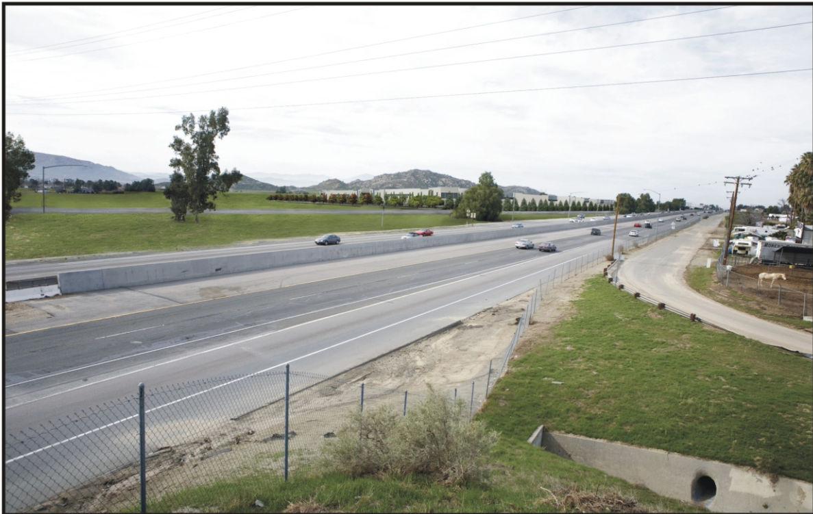
Project Buildout Condition
