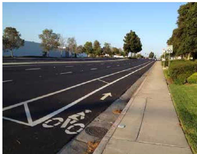
Buffered bicycle lane - San Diego, CA
