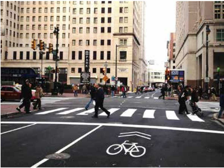
13B) Shared lane marking directing cyclists through intersection - Philadelphia, PA
