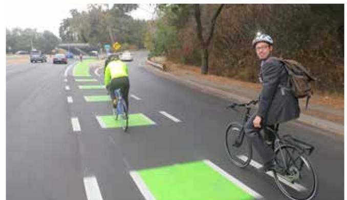
Green transition lane - Alpine Road at I-280, San Mateo, CA
