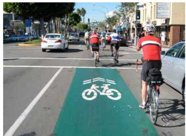
4B) Shared lane markings or "Sharrows" remind vehicle drivers to expect cyclists and help cyclists to properly place themselves within the roadway away from parked car doors. On streets with very high bicycle volumes, both purposes can be enhanced by supplementing markings with green paint - Oceanside and Long Beach, CA
