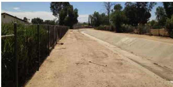
Typical flood control channel
