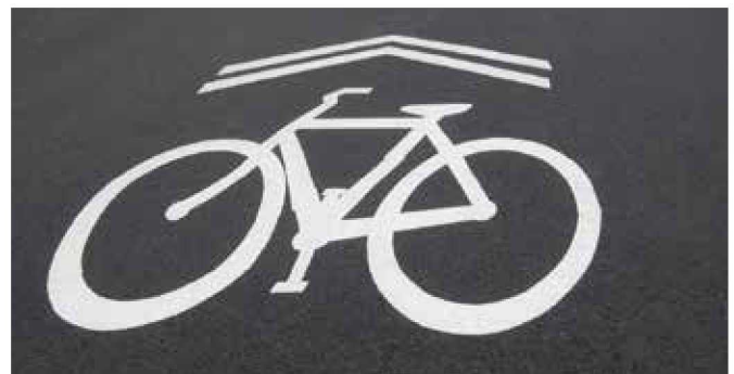
Shared lane marking (“Sharrow” or “SLM”)
