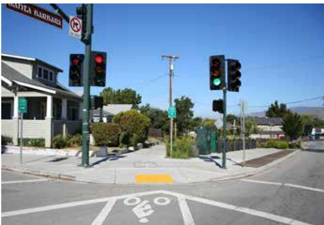
Bicycle boulevard/roadway intersection treatment with signalized diagonal bicycle crossing - San Luis Obispo, CA
