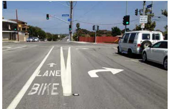
11B) Bicycle lane properly installed between through travel lane and right-turn-only lane - Huntington Beach, CA
