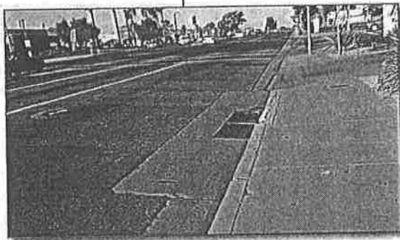
PHOTO 5 | Inserts and filters to existing and new catch basins are recommended
