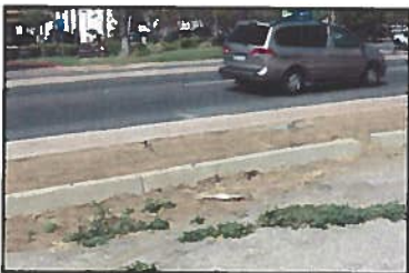
Unmaintained public right-of-way and weeds in parking lot.
