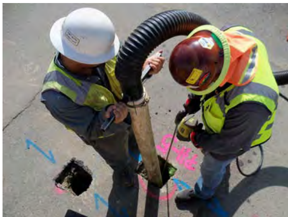
C Below technicians performing potholing
