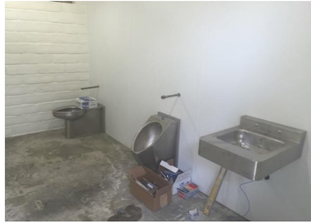
Park Restroom Renovations
