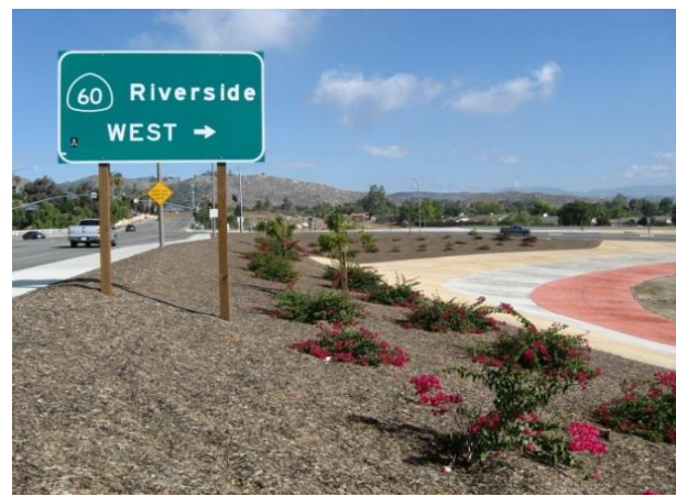
SR-60 / Nason Street Overcrossing Bridge (Landscape Establishment)
