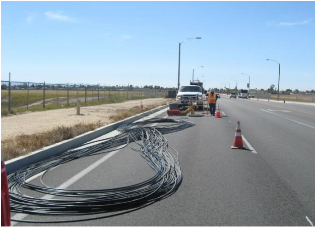
Citywide Fiber Optic Communications Expansion
