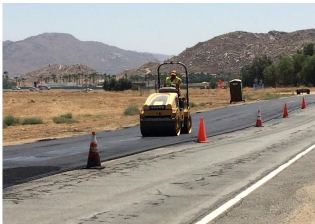
Pavement Rehabilitation Program
