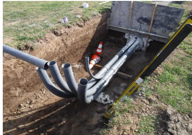
Feeder Line Trenching
