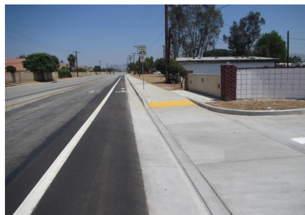
Pedestrian Ramp Improvements
