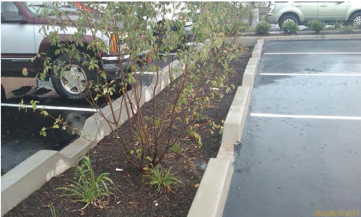
Figure 5-35 Example of Bio-swale
