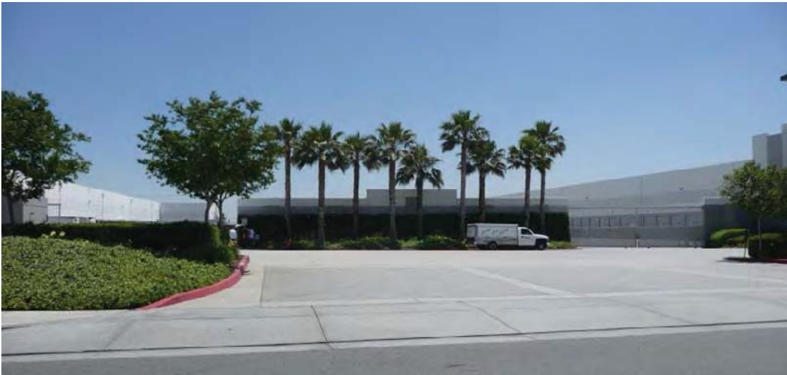
Figure 5-25 Example of Appropriate Ground Mounted Equipment Screening
