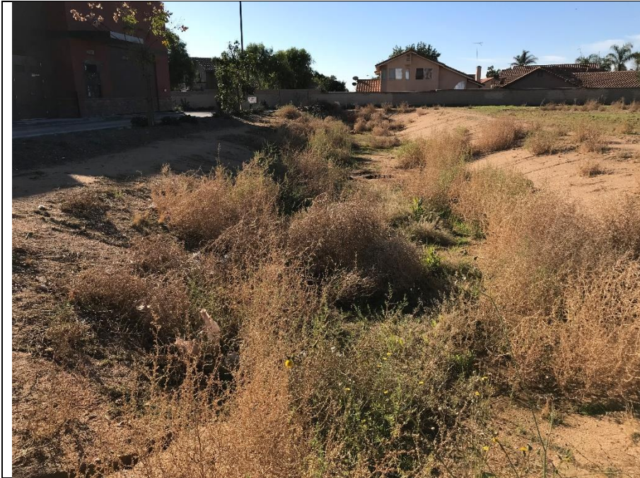
Photo 5. Detention basin located in southwest corner of project. Plant growth evident
