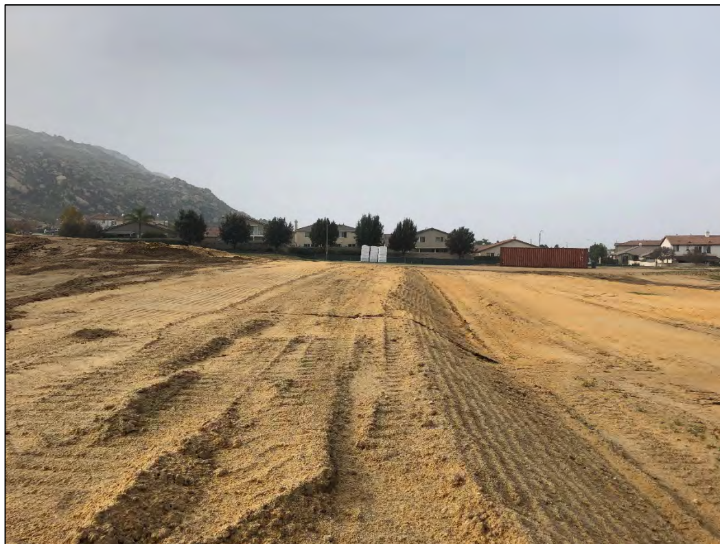
Looking west at the Project Site.
