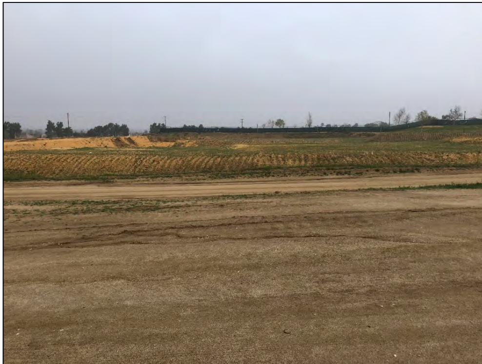
Looking east across the Project site at the previously graded development pads.
