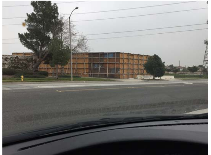
K-Rail Plywood & Acoustic Material
