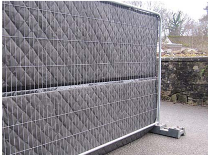
Temporary Fence & Acoustic Material 01
