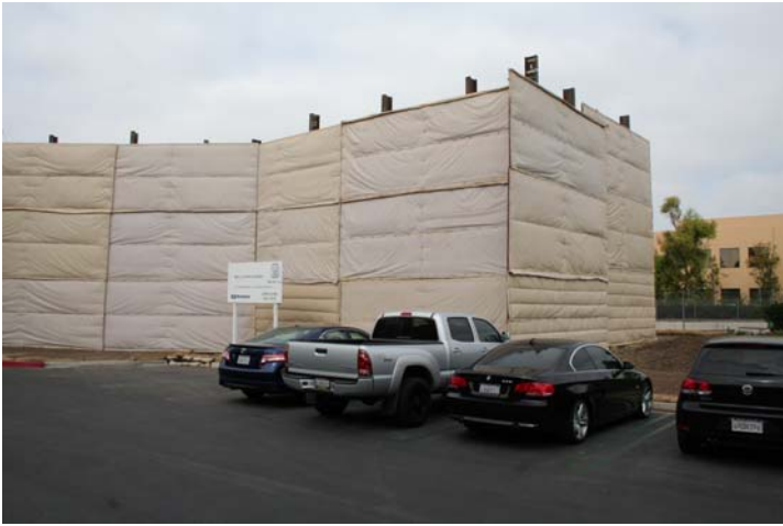
I-Beam & Acoustic Material 01
