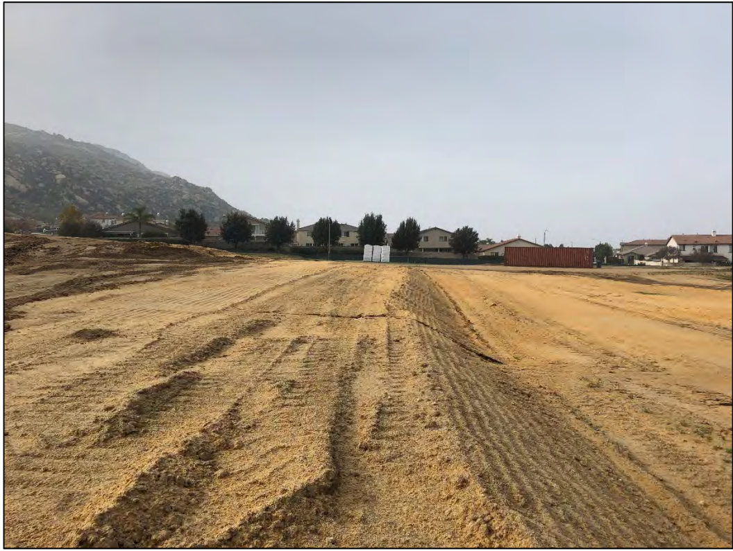
Looking west at the Project Site.
