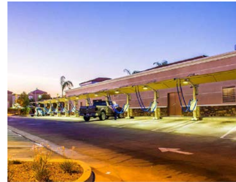
REPRESENTATIVE PHOTO OF THE PROPOSED SYSTEM WITH FABRIC CANOPY 04 CARWASH VACUUMS SCALE: NTS
