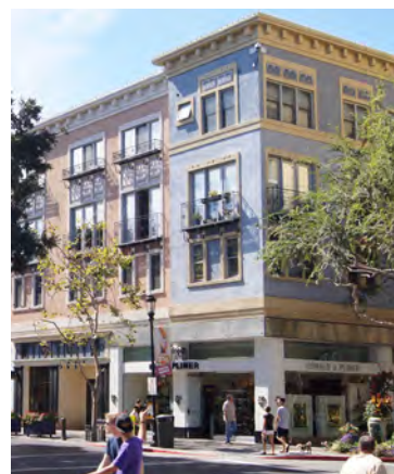
Transit-oriented development, San Jose, CA
