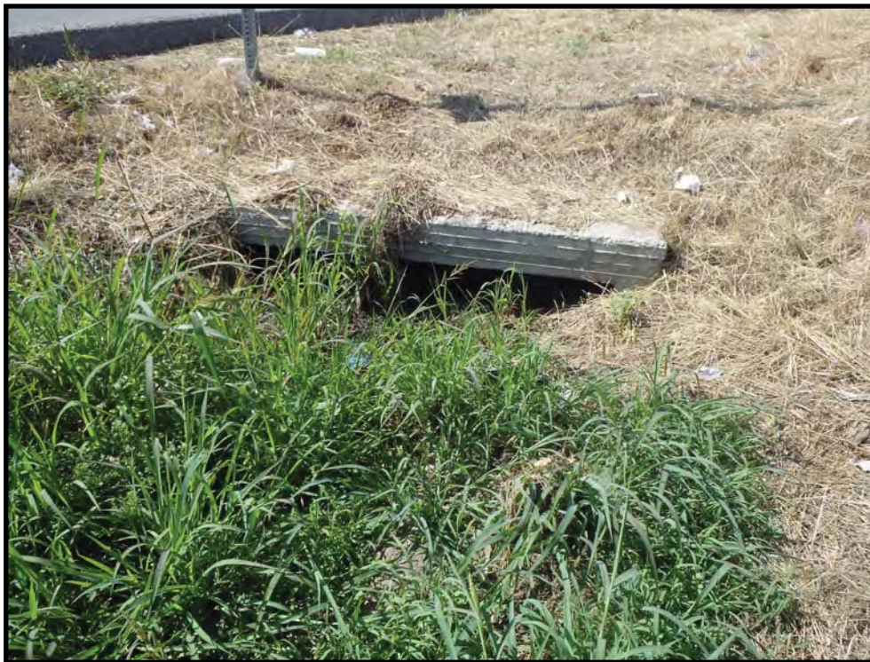
PHOTOGRAPH 1 - The onsite, ephemeral drainage feature (D1) is fed from a storm drain outlet at the northwest corner of the Project Site and flows south.
