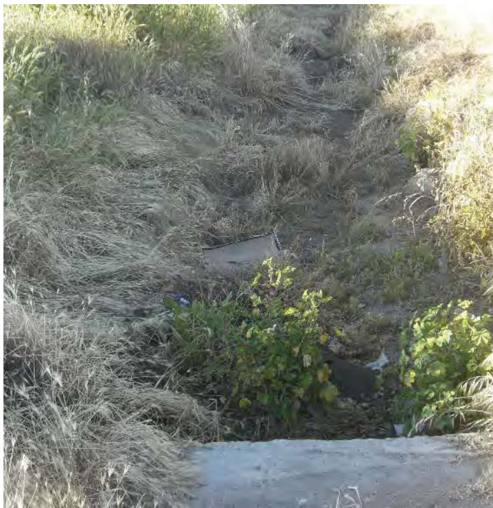
Photograph 6: Project Site's ephemeral drainage ditch, view towards the south
