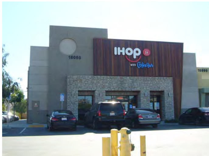
5) View of the adjacent IHOP restaurant to the southwest.
