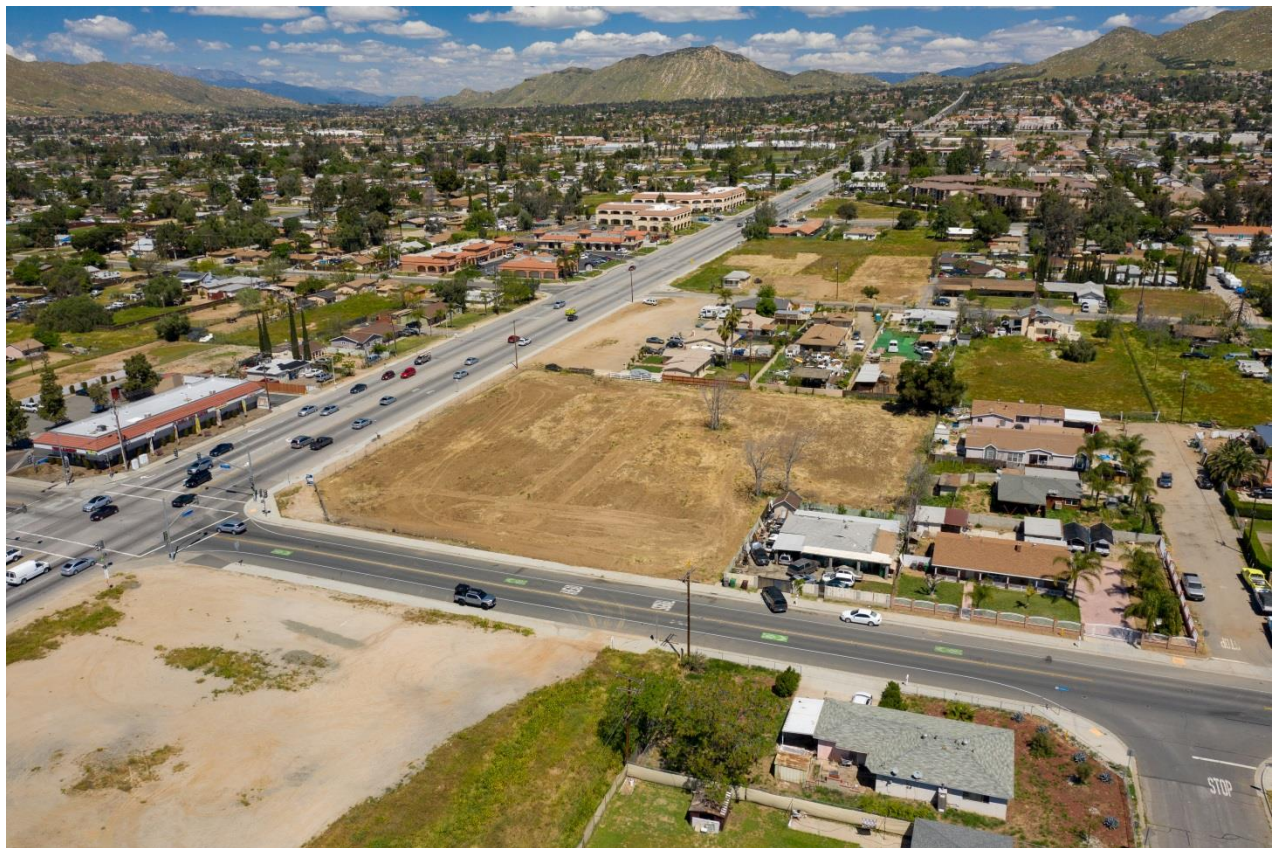
Photograph 2. Aerial view of project site, facing northwest.
