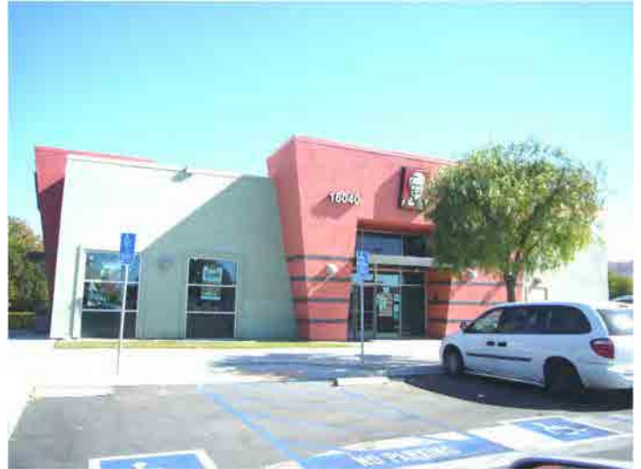
6) View of the adjacent KFC restaurant to the southwest.
