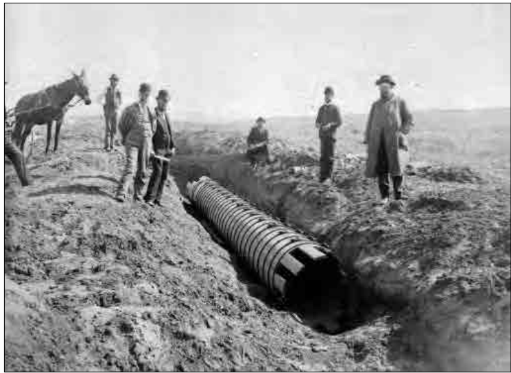
Figure 5. Frank Brown, far right, during pipeline placement, circa 1891 (Ghori 2014)
