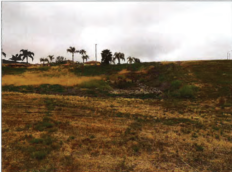
Photograph 3: View of culvert located on the southwestern side of The Rancho Belago Phase II Site. View to the southwest.
