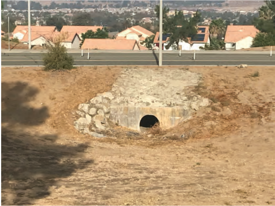
Photo 5 Cement culverts at site
