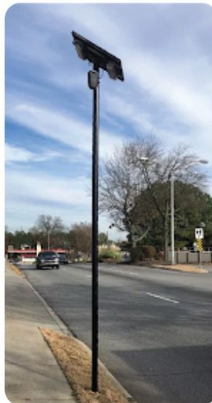
Entrance to Hotel Solar & Flock 14 foot pole
