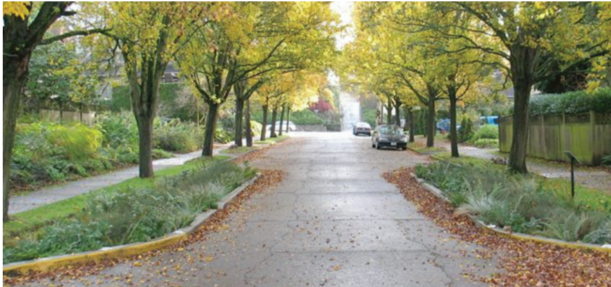
Street trees can be placed at pinchpoints to further narrow the profile of the roadway. Source: NACTO
