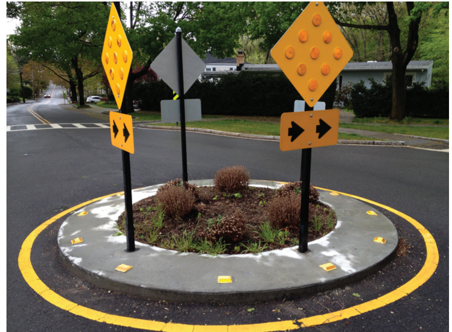
Mini roundabouts can be placed on low traffic volume residential streets. Source: NACTO
