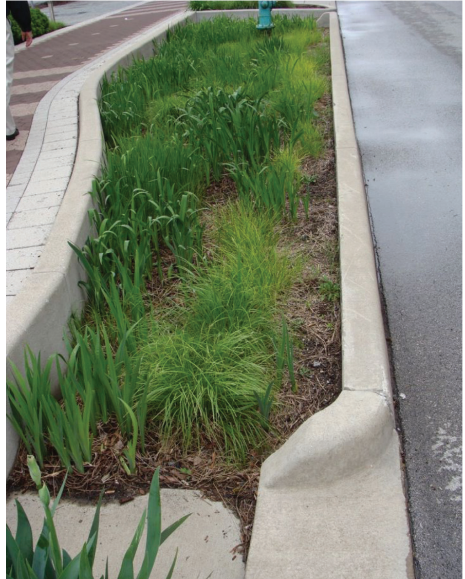
The use of bioswales can assist with stormwater management by reducing stormwater runoff. Source: NACTO
