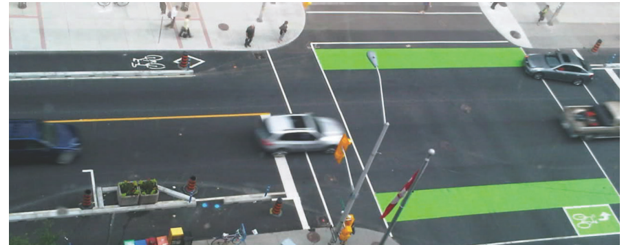
Two stage left turn lanes prevent motorists from turning into bicycle turn lanes. Source: NACTO
