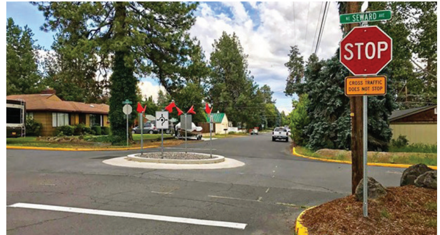
Orienting stop signs away from the greenway minimizes bicyclist delay. Source: City of Bend
