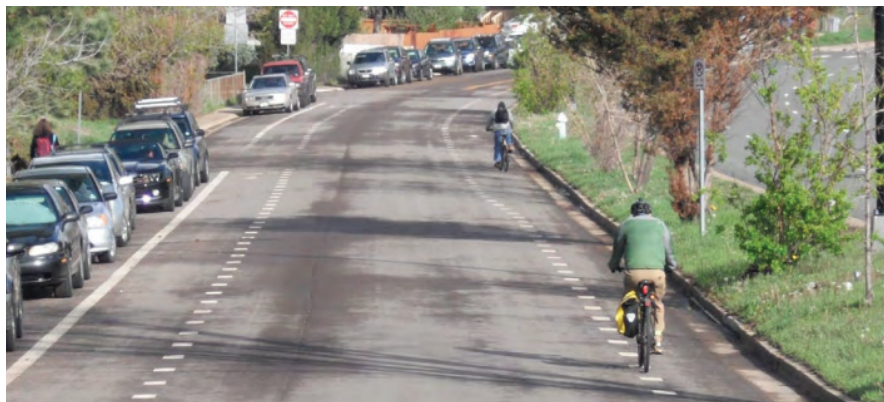
Advisory bike lanes in Boulder, CO can provide bicyclists a safe connection where there is not sufficient space for a traditional bike lane. Source: City of Boulder
