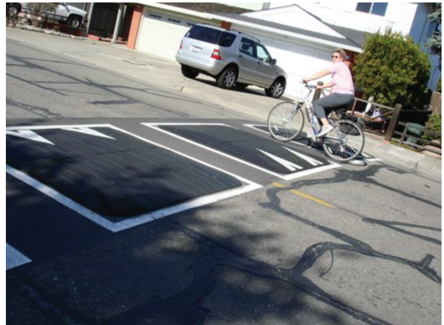
Speed cushions can be designed to provide speed reducing effects to motorists without interfering with bicyclist connectivity. Source: NACTO
