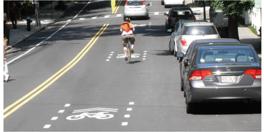
Shared lane marking on a residential street in Brookline, MA provide bicyclists right of way on low traffic volume streets. Source: NACTO
