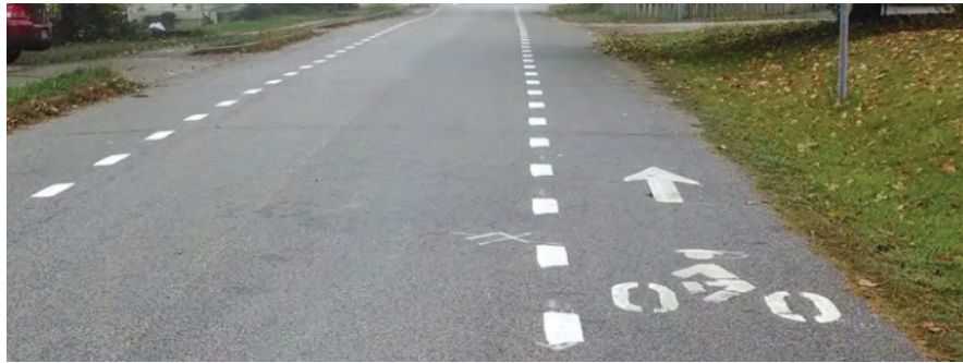
Advisory bike lanes in Bloomington, IN create a visual narrowing of the roadway. Source: Scott Robinson, City of Bloomington
