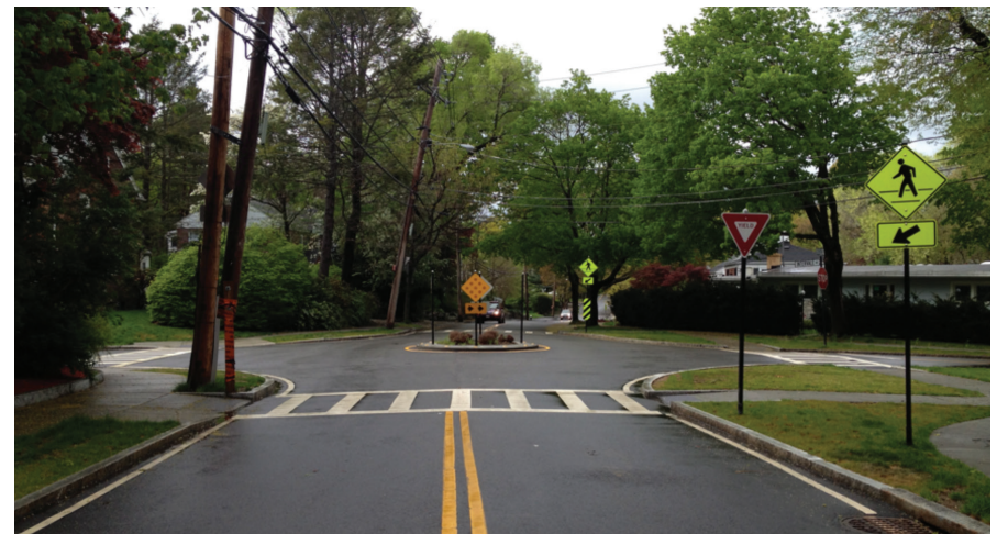
Mini roundabouts have been shown to reduce traffic speeds at uncontrolled intersections. Source: NACTO
