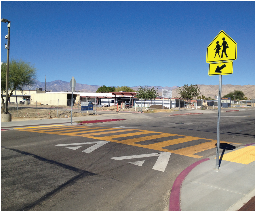
Raised crosswalks maximize visibility of pedestrian crossings. Source: KTUA
