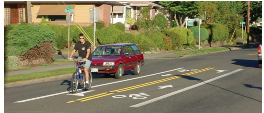
A center left-turn lane in Portland, OR allows bicyclists to turn left from the cross street back onto the greenway. Source: NACTO
