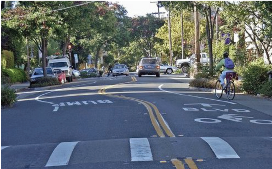
Chicanes can slow traffic speeds considerably on low traffic volume streets. Source: NACTO
