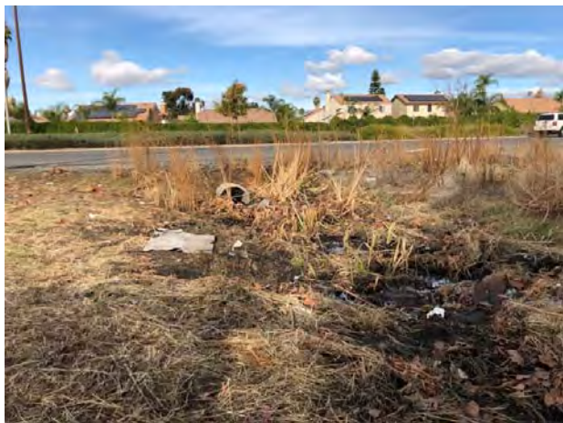
7.View of the storm water easement drain on the northeast.
