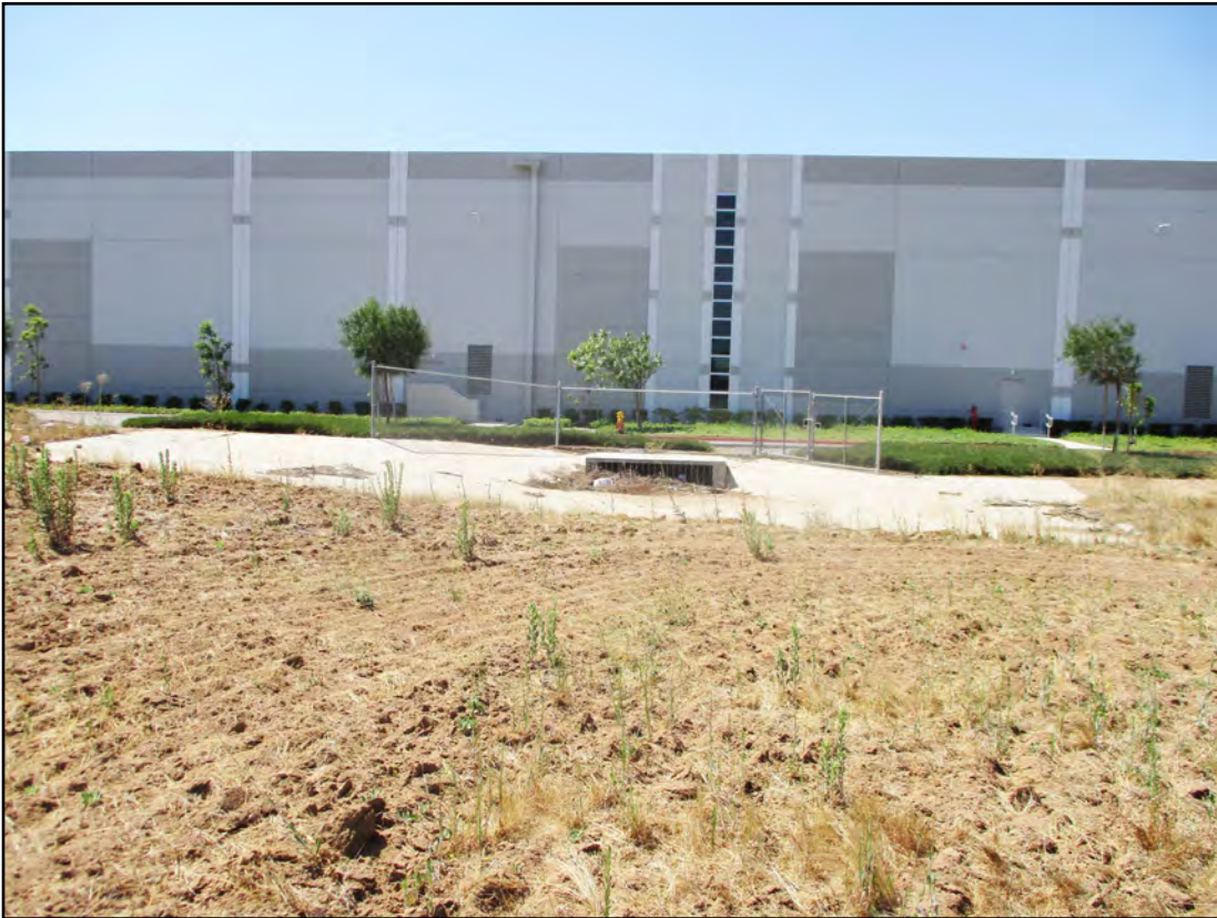
Photograph 2 - Southward view of down drain located at end of the end of Drainage A
